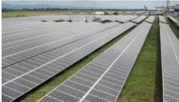
Captive Solar PV Plant & Solar Roof Tops
